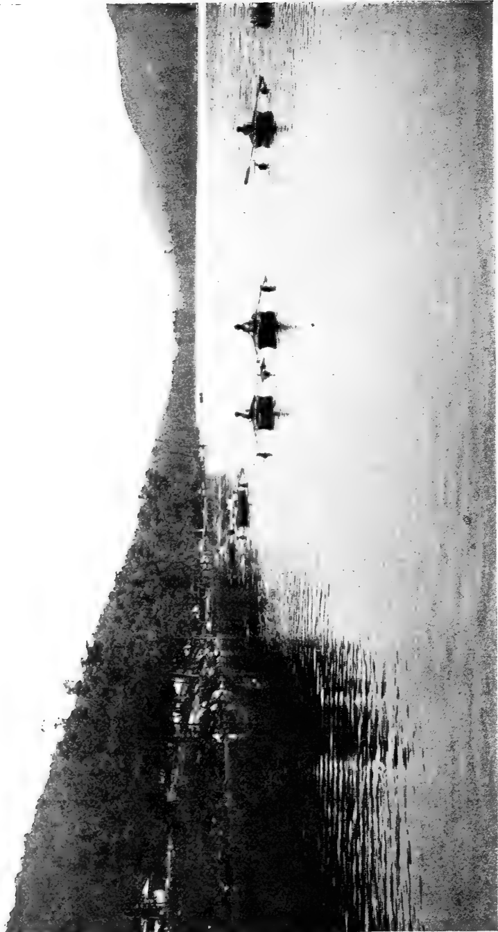
Fig. 19. Applying copper sulphate treatment to Carr Pond. The copper sulphate is suspended in loose-meshed bags at the rear of the rowboats.
